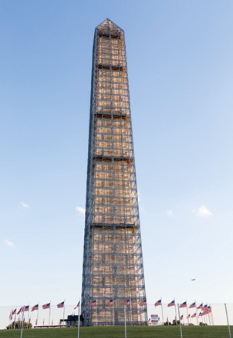
The Washington Monument encased by scaffolding for earthquake damage repairs.
