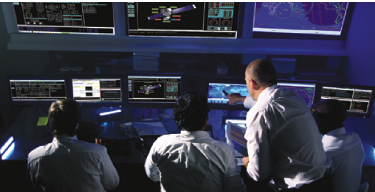
A network operations center — photo is courtesy of Kratos Defense.
