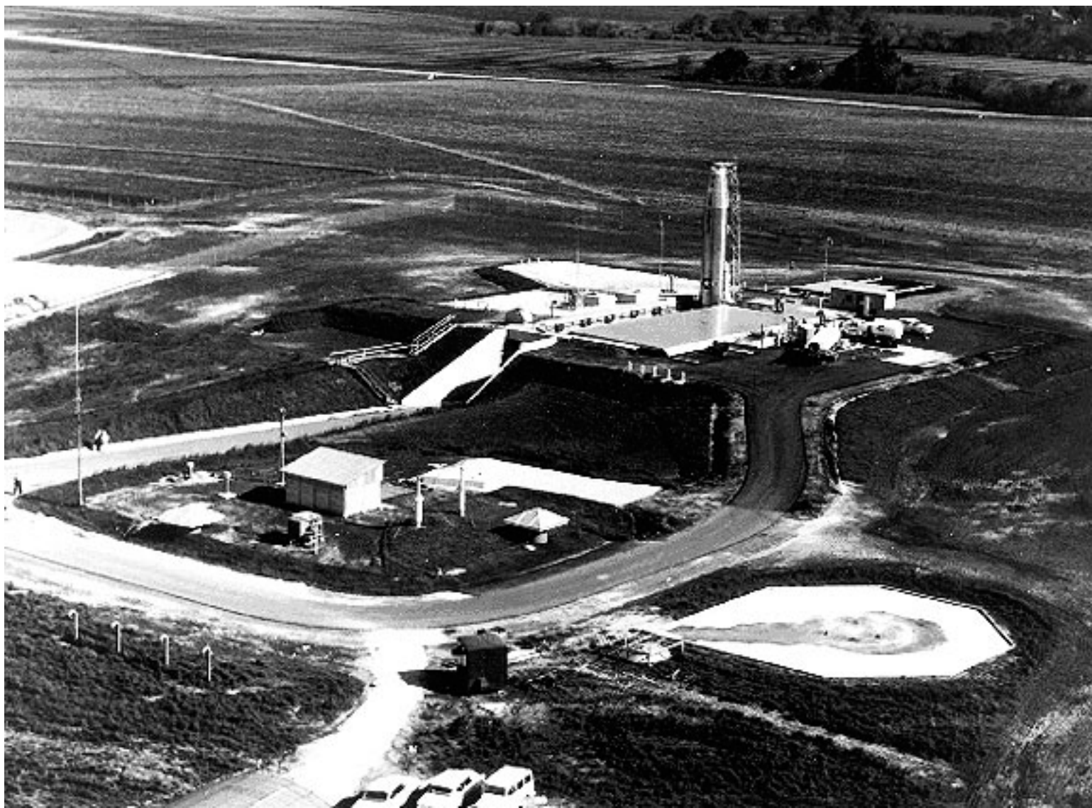
An Atlas E missile at its launch facility. The square ventilators in the photo's foreground indicate the location of the underground launch control and command.
