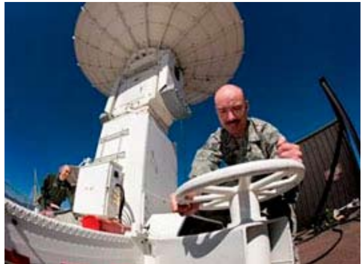
Master Sgt. Eric Gemmell adjusts the support system of a Transportable Antenna System while Capt. Joseph Fixemer directs the leveling of the system. The antenna is a component of the Rapid Attack Identification Detection Reporting System, or RAIDRS, at Peterson Air Force Base, Colo. RAIDRS is the new defensive counterspace weapon system for 2010.
