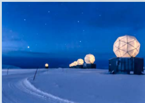
Photo of the Iridium ground Station, courtesy of Ivar Stakvik.
