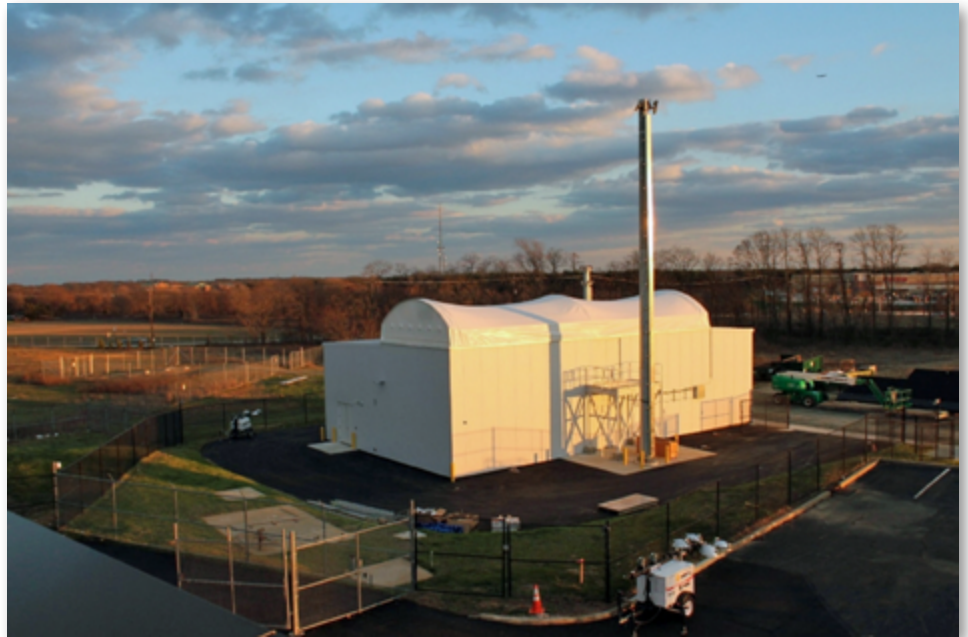
The Space Fence testing facility is representative of the larger Gallium Nitride (GaN)-based digital array radar system under construction on the Marshall Islands. This innovative system will transform the way the United States Air Force monitors thousands of orbital space objects. The photo is courtesy of Lockheed Martin.
