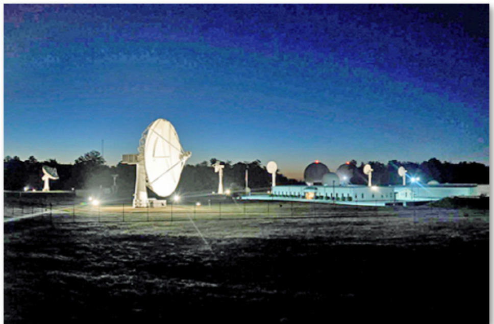
The Blossom Point Tracking Facility (BPTF) campus, located 35 miles south of Washington, D.C., consists of a satellite mission operations center, multiple antennas, and an existing infrastructure capable of providing space system command, control, and management for all customer classes. The facility, operated by the US Naval Research Laboratory, is in continuous 24 hour, 7 day operation and at present supports numerous on-orbit spacecraft. Photo is courtesy of NRL, Jamie Hartman.
