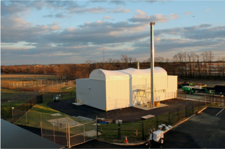
The Space Fence testing facility is representative of the larger Gallium Nitride (GaN)-based digital array radar system under construction on the Marshall Islands. This innovative system will transform the way the United States Air Force monitors thousands of orbital space objects. The photo is courtesy of Lockheed Martin.
