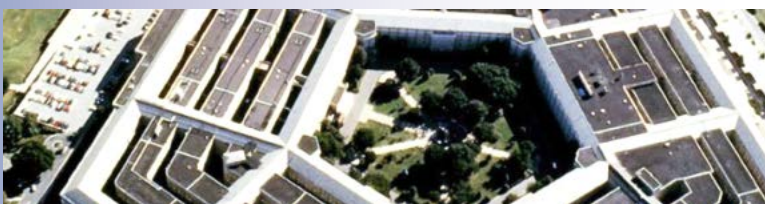
The Defense Information Systems Agency's (DISA) Defense Information Systems Network (DISN) serves all branches of the military services, the executive branch, the combatant commands, 14 DoD agencies, and nine field activities.
