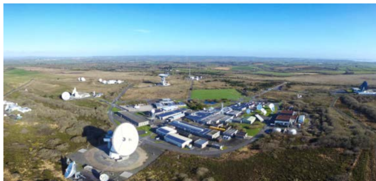
Goonhilly Earth Station.
