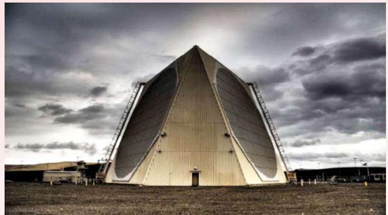
The 7th Space Warning Squadron has an enhanced Upgraded Early Warning Radar system with a greater capability to detect and track missile attacks against the U.S. and its allies, at Beale Air Force Base, California. (U.S. Air Force photo)
