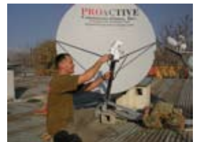
Jon Sintel, PCI Engineer, handling the installation in Bagram, Iraq
