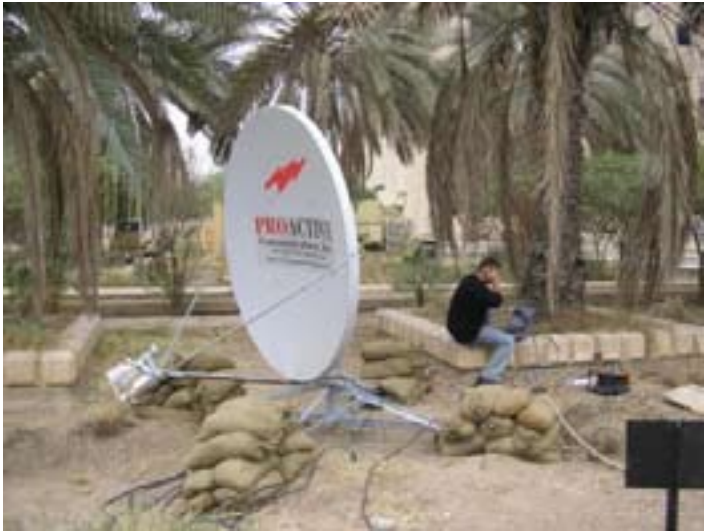
Ali Installing IC2N Site in Baghdad
